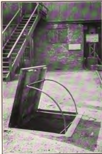
PLATE 15.—PROTECTIVE DEVICE FOR TRAP DOORS
